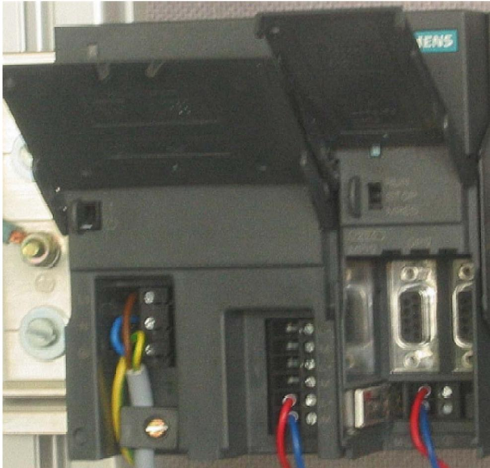
Figure 5-1 Wiring the power supply and the CPU
